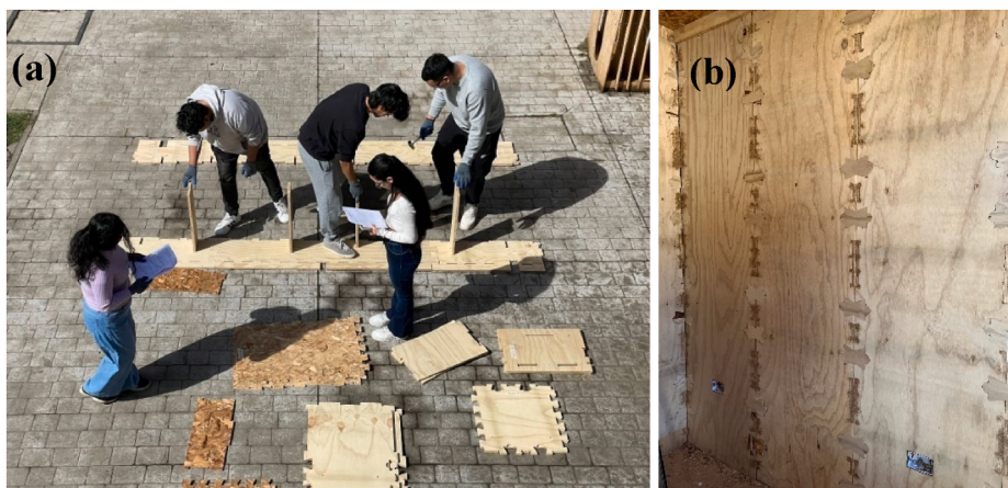
Fig. 7. Student group in the process of wall assembly (a) and installation in laboratory prototype (b).
